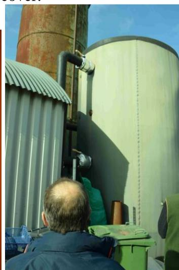
**990kW Heizomatt boiler (orange) with fuel silo to left Outdoor Buffer Tank**
