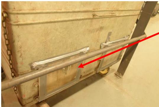
**Ash bin air leakage.** Due to bad design, the ash bin access gates at the base of the bins are buckled and allow air to be sucked in to the main boiler combustion area. This will cause turbulence, and a mixing of air temperatures leading to inefficiencies of controls. A simple fix ensuring a good seal was being installed in late February 2020. It will likely lead to a further 2-3% efficiency improvement.
